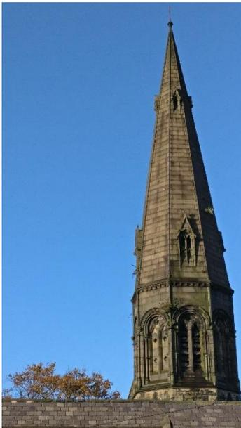
**Spire:** scaffolding will be erected from 12<sup>th</sup> March onwards and the building work will commence afterwards, with this first phase of our building project expected to be completed by 8<sup>th</sup> June. The work involves taking down and re-fixing the top of the spire, installing a new finial at the top, re-pointing most of the tower and spire, and installing pigeon-proof barriers on the windows. We are hoping to share photos of progress, as well!
